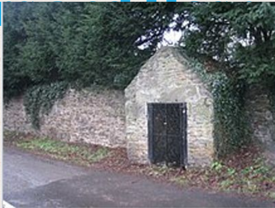
St. John's Well The Victorian well house over the medieval well [1]
